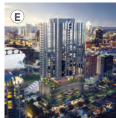
70 Rainey 70 Rainey St 160+ RESIDENTIAL UNITS | 35 STORIES 70raineycondosaustin.com
